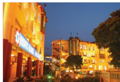
DURGAPUR CITY CENTRE DURGAPUR
