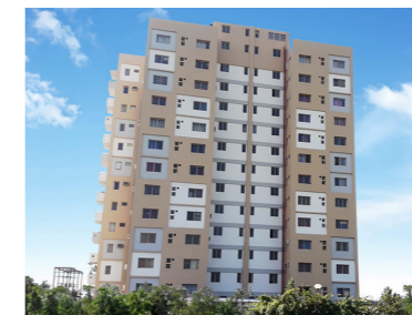
The Arena, Haldia International Sports City, Haldia
