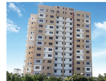
The Arena, Haldia International Sports City, Haldia
