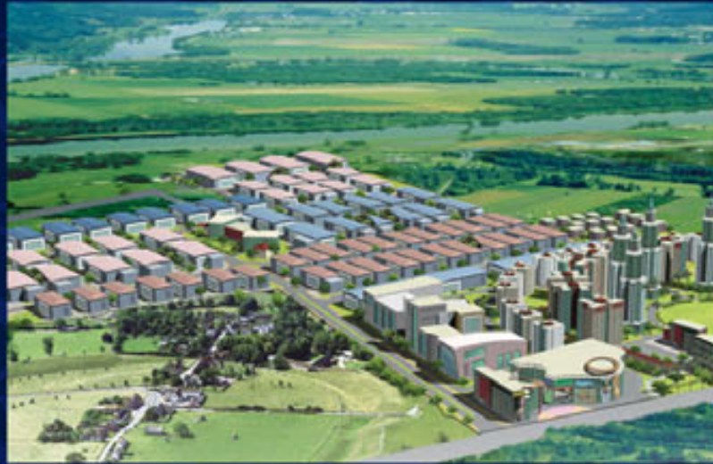
Integrated Industrial Park, SILIGURI, WEST BENGAL
